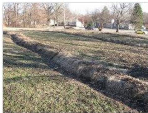
A simple infiltration swale can reduce runoff and trap water on a sloped site.
